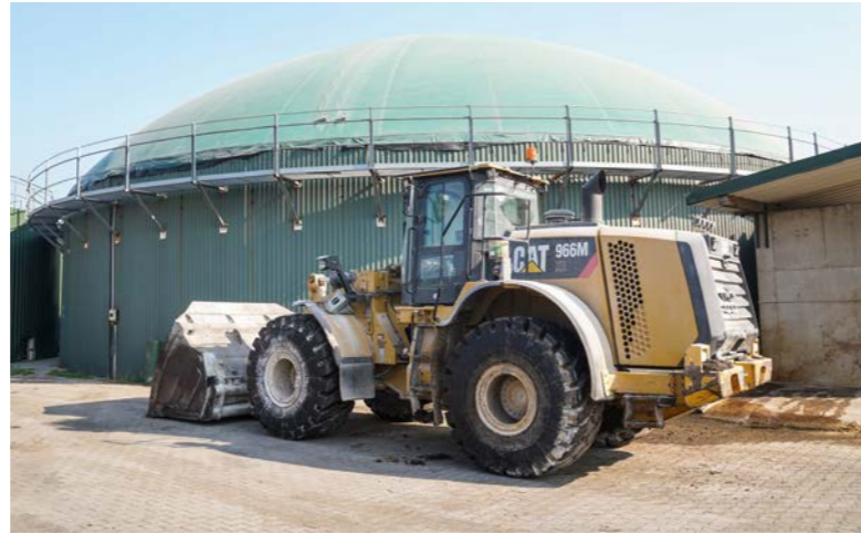
Plenty of throughput: The biogas plant has an operating permit that allows it to ferment 45,000t of biomass.
