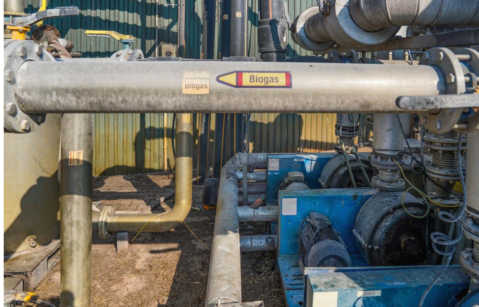
Its own gas network: The biogas generated by the plant is distributed to various co-generation units in the district of Recke.
